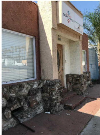
Foundation for Second Chances Building
