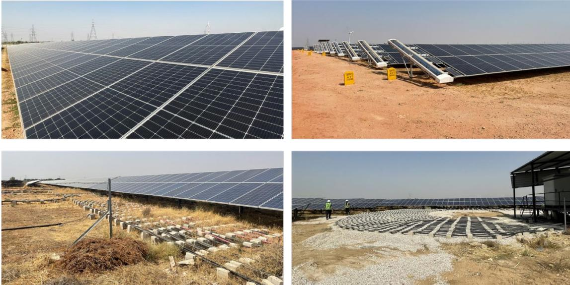
*Photo 3: The top two photos represent solar fields with buried cables and well-groomed grounds. The bottom two photos represent solar fields with above ground cables and unkempt grounds, which can increase the potential for hazards.*
