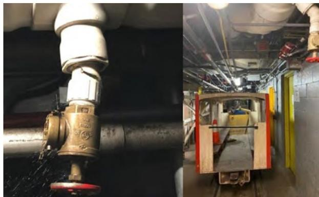
*From left to right: cracked low point drain; train passenger cart. (U.S. Navy photos)*
