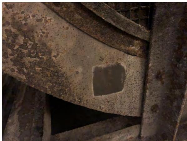
**Figure 19. AHU Intake with Lead Residue**
