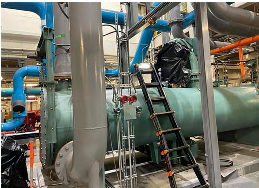
**Chiller #1 exhibits excessive bearing wear and the chiller plant is nearing the end of its life expectancy.**
