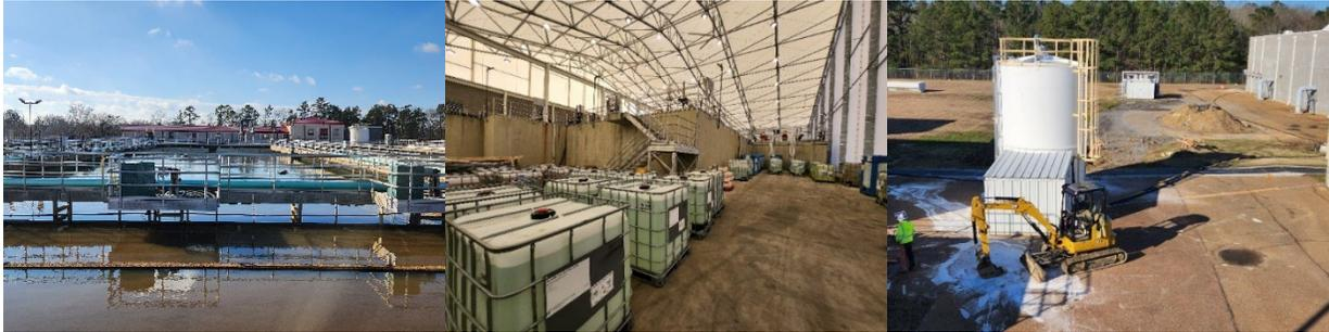
Left to right: O.B. Curtis conventional water treatment, liquid soda ash storage and membrane treatment, and external liquid lime treatment tank. (EPA OIG images)
