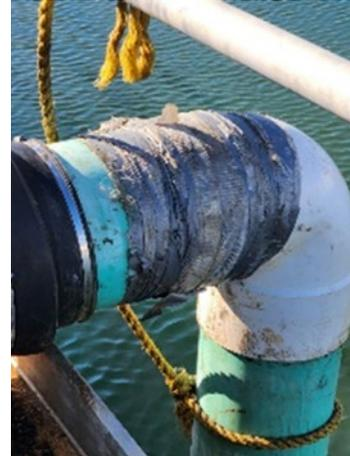
Example of poor maintenance of pipes using duct tape at the traditional side of the OB Curtis plant. (EPA OIG photo)
