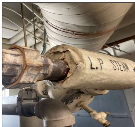
Figure 2. Damaged Asbestos-Containing Cement Pipe Wrapping in Mechanical Room 6607 5
