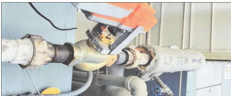
Figure 2. Damaged Asbestos-Containing Cement Pipe Wrapping in Mechanical Room 6607 5
